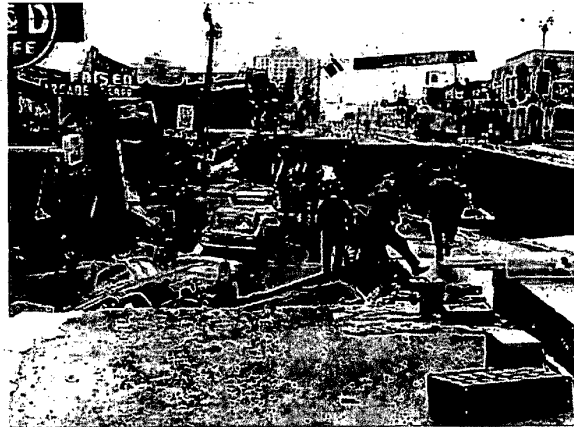
Fig. 3 Collapse of Fourth Avenue, Anchorage, Alaska, at the head of a 15 ha block slide triggered by the M8.3 Alaska earthquake of 27 March 1964 (Photo by US Army)
