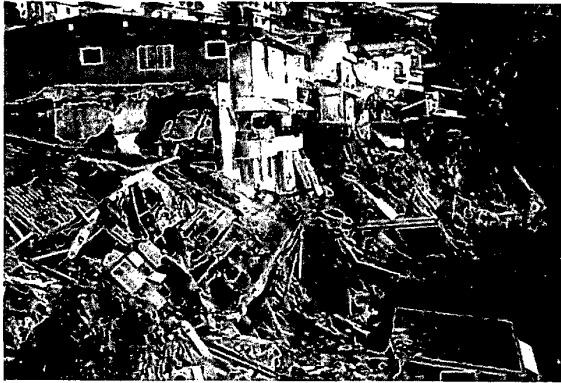
Fig. 12 Homes in high-cost residential area of Caracas, Venezuela, that were destroyed on 29 September 1993 by a rainfall-triggered landslide (Photo by D. A. Salcedo, Universidad Central de Venezuela)
