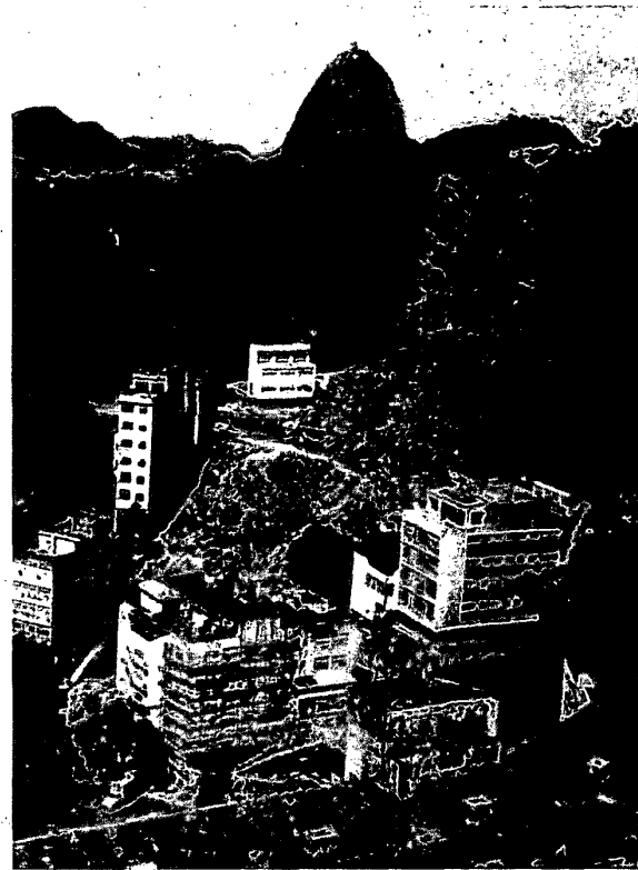
Fig. 4 The 18 February 1967 Bairro Jardim-Laranjeiras landslide, Rio de Janeiro. This landslide resulted in the destruction of two apartment buildings and the deaths of 110 people (Da Costa Nunes et al. 1979) (Photo by Ruy Macial, Geo-Rio, Rio de Janeiro)
