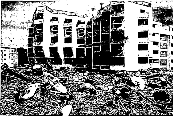
Fig. 14 December 1999 debris flow damage to the city of Caraballeda, north coast of Venezuela (Photo by L.M. Smith, Waterways Experiment Station, U.S. Army Corps of Engineers)
